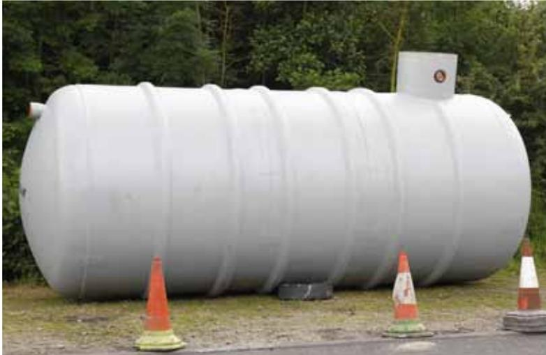
When the outflow of water and oil from a wash bay enters the wash bay interceptor the oil becomes emulsified due to detergents and hot water. Because the water is no longer free flowing, a standard wash bay interceptor will not separate the oil which would simply pass through the chambers.
